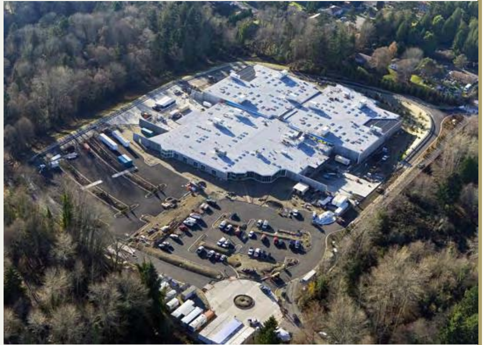
SCORE Jail, South Correctional Entity - Des Moines, Washington Architect: DLR Group
