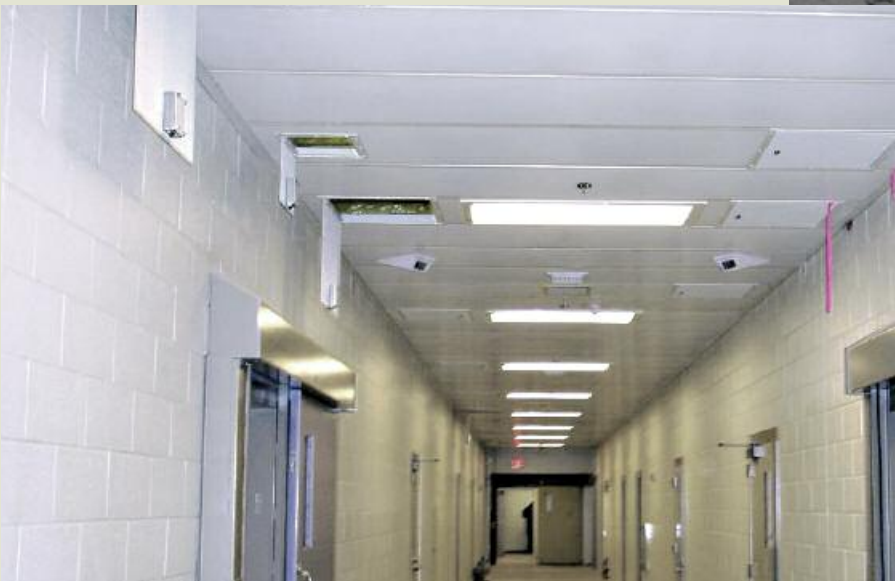
BarrierDek Single Skin Metal Plank Ceiling
