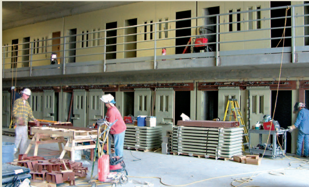
TrussWall construction site - walls erected after building is enclosed
